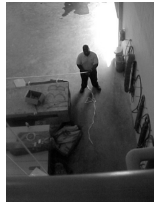
Figure 6: Hoisting the weight
